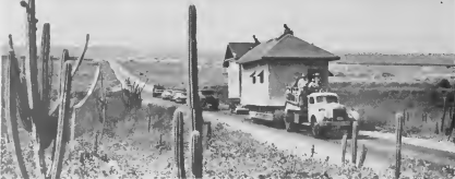
FOLLOWED BY a line of early-morning traffic, the former Acid & Edelcaan Plant office building section No. 1 moves slowly over the Santa Cruz road toward its new home at Imeldahof. SIGUI PA un linea di trafico mainta tempran, e anterior oficina di Acid & Edelcaan Plant, seccion No. 1, ta move lentamente over di camina di Santa Cruz pa su sitio nobo na Imeldahof.
